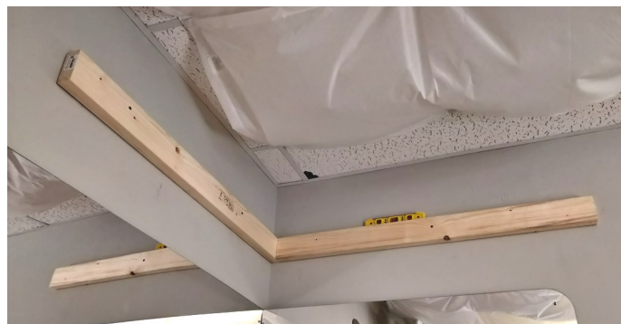
2x4's installed and ready for the Corner Shower
